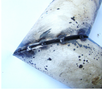
Figure 9.23: Tack Welding of L Elbow
